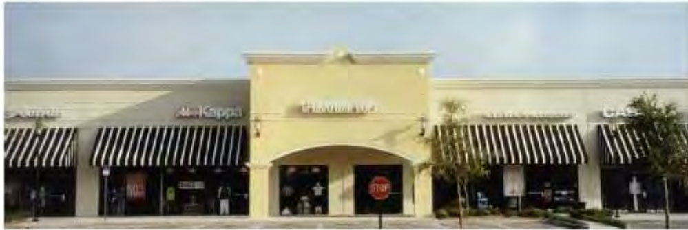
Figure 27. Example Building Entrance Enhancement
