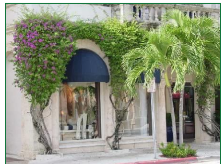
Figure 44. Planters Adjacent to Buildings
