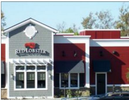
Figure 37. Rooftop Units Screening
