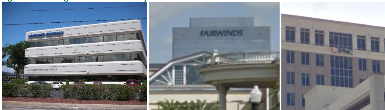
Figure 48. Wall Sign Above Second Story
