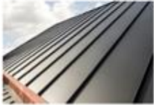
STAIR COLUMN ROOF
