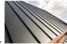
STAIR COLUMN ROOF
