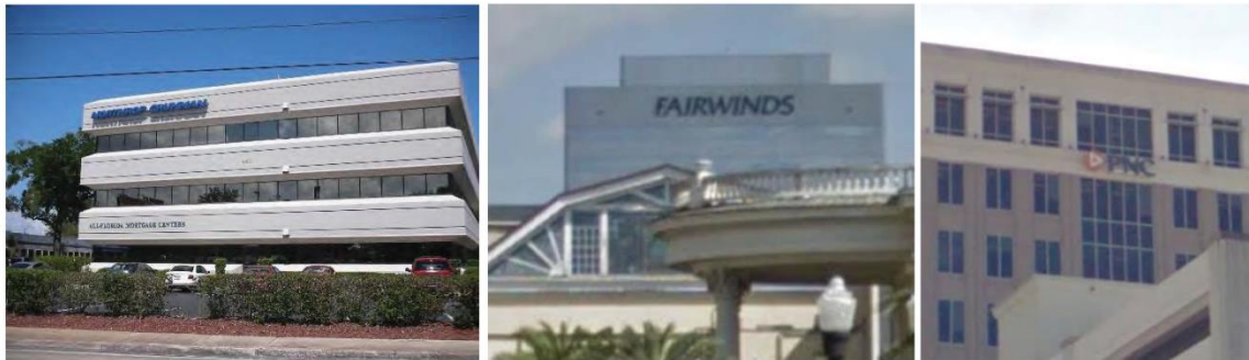
Figure 49. Wall Sign Above Second Story
