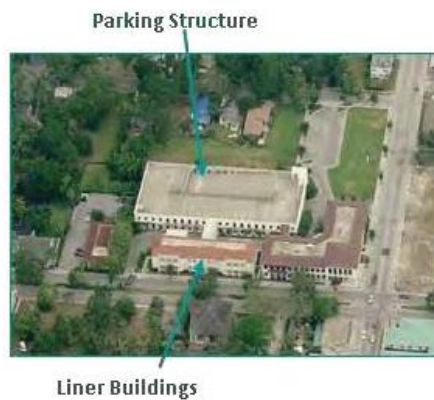
Figure 18. Detached Liner Building
