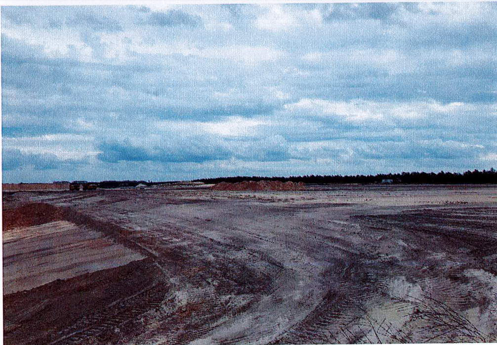
(2) View of Subject Looking East from West Property Line. Photograph taken on December 10, 2023, by Edwin R. Barfield
