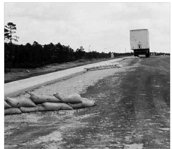
Figure 3.5j. Curb inlet gravel filters
