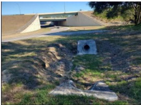
Image 2: Existing Stormwater Conveyance
